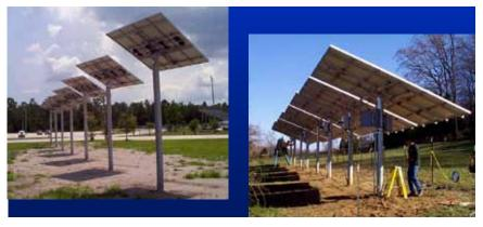
Figure 23. Pole-mounted arrays use either fixed, adjustable, or sun-tracking arrays installed on a rigid metal pipe.
