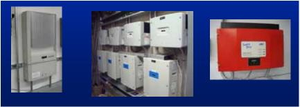
Figure 73B. String inverters are small inverters in the 1 to 12 kW size range, intended for residential and small commercial applications.
