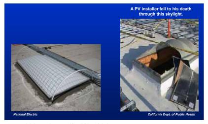
Figure 85. Skylights must be protected from fall hazards by barriers or covers.
