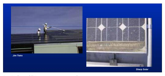
Figure 114. Cleaning soiled PV arrays is a common maintenance need.
