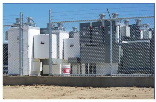
Figure 74. Utility-scale inverters use higher DC input and AC output voltages to reduce losses, and the size and costs of the conductors and switchgear required.
