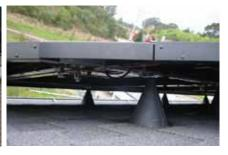
Figure 21. Standoff mounts are the most common way PV arrays are attached to sloped rooftops.
