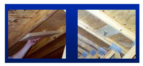
Figure 106. Additional blocking may be required for some installations to adequately secure point attachments to the structure.
