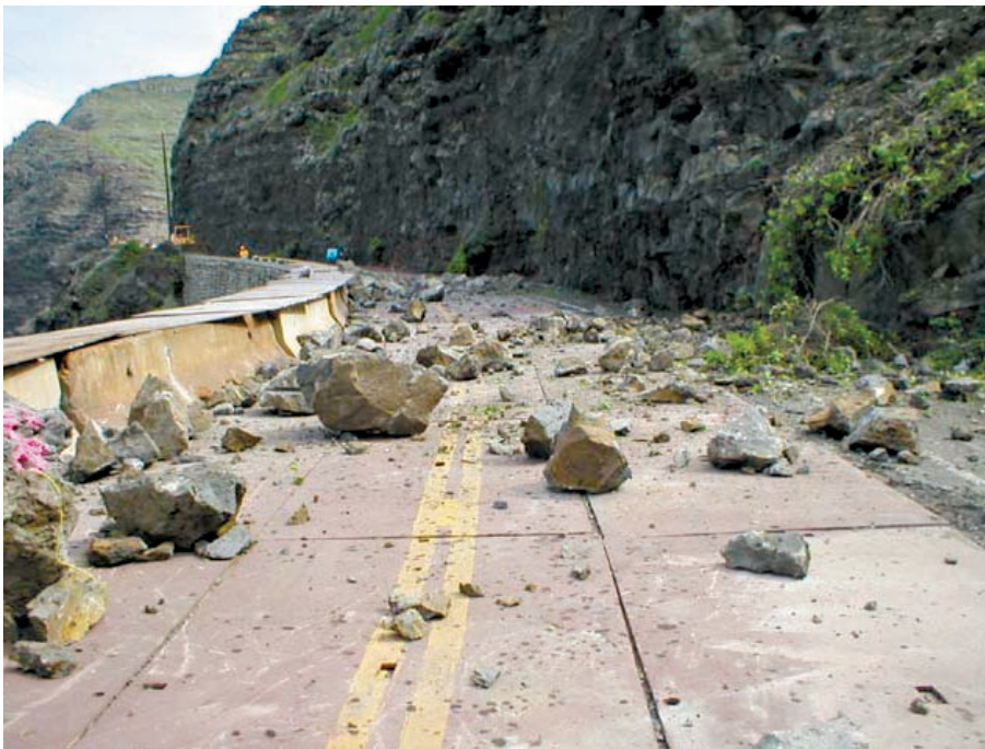
Figure C29. Rocks dislodged by scaling and blasting. (Photograph by Washington Department of Transportation, USA.)
