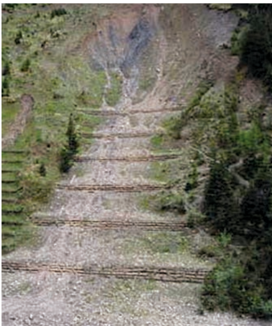
Figure C7. Schematic and photograph of a crib wall check dam, which is one kind of check dam. (Graphic from Reference 11, photograph taken in Trafoi, Italy, courtesy of "Erosion Control," Forester Communications, Santa Barbara, California, USA.)
