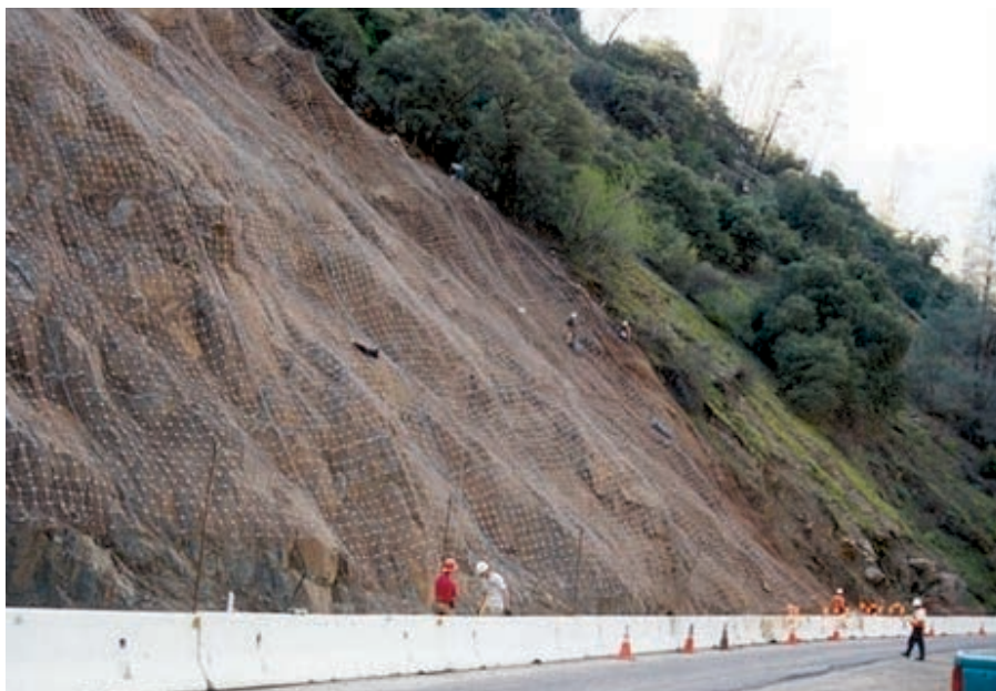
Figure C21. Example of wire mesh placed over a rocky slope to contain the rocks that may come down.
