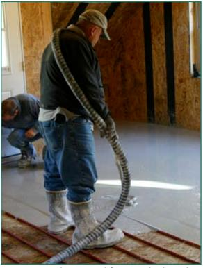
Gypcrete poured onto second floor provides thermal mass for radiant heat tubing
