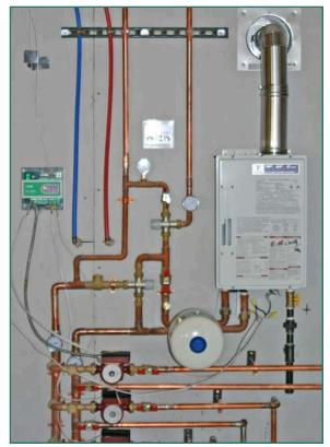
Wall mounted tankless heater that provides domestic hot water and space heating for a 2,400 square foot building
