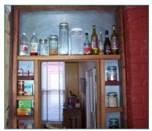
Sheet metal used for open shelf backing
