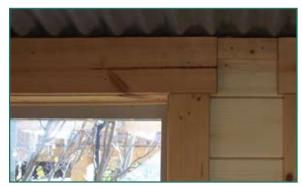
Butt jointed 1-inch standard pine boards used as window casings
